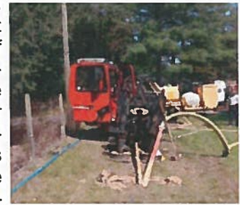
Trenchless Replacement of Line
